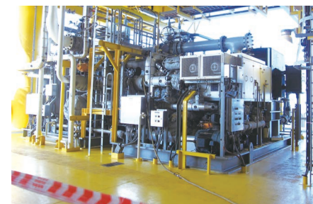
Vapor Recovery Compressor - Vietnam Offshore 3225MMC / 600kW
