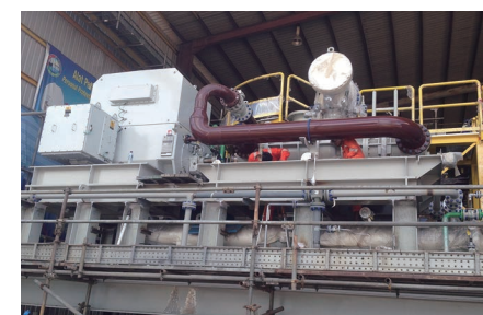
Gas Chiller - Africa Offshore 4032XLLL / 2400kW
