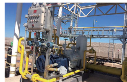
LPG Transfer Compressor - Mexico 6HK / 45kW
